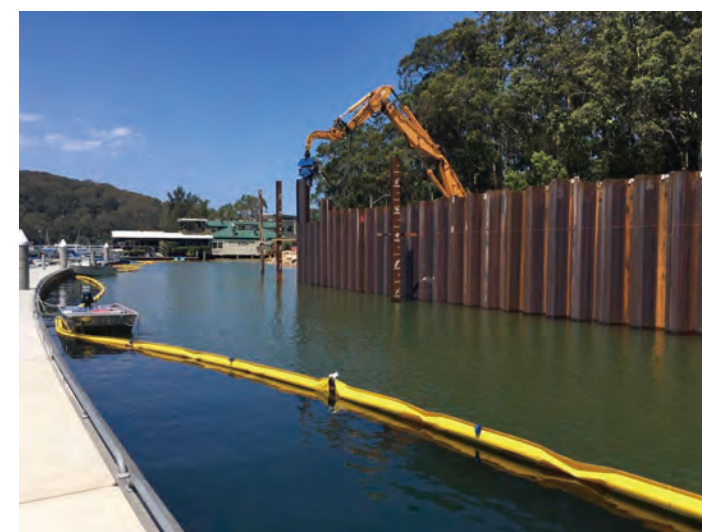
Hat-type Sheet Pile Church point seawall / Australia
