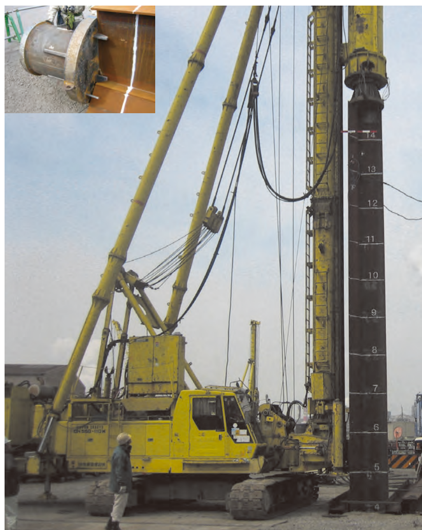
Driving of a Hat+H sheet pile
