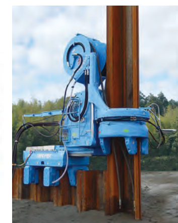
Pressing-in of Hat-type sheet pile
