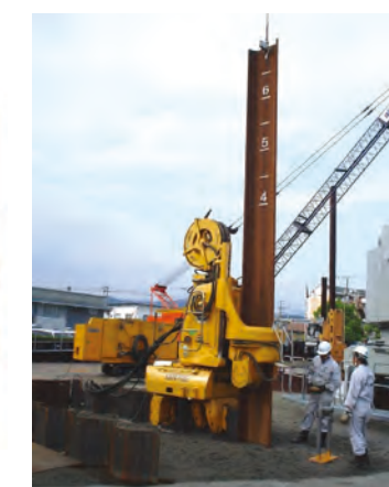
Pressing-in of U-type sheet pile
