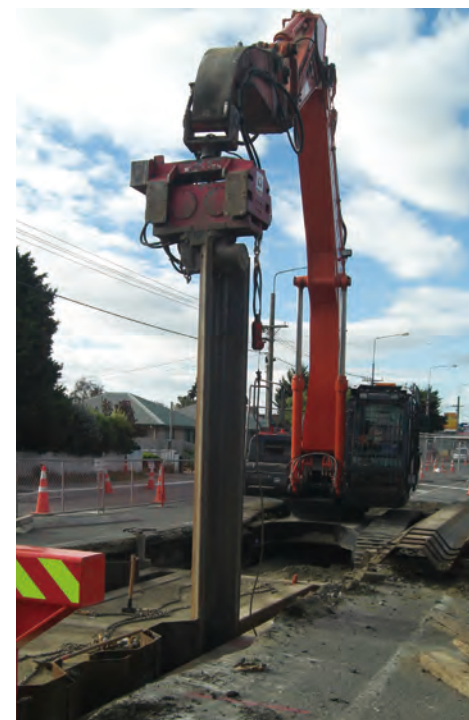
Driving of a Hat-type sheet pile
