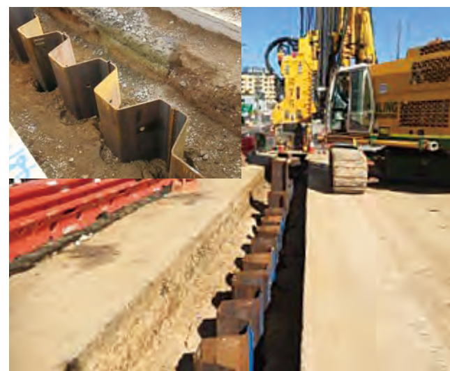
Hat-type Sheet Pile O-Bahn City Access Project / Australia
