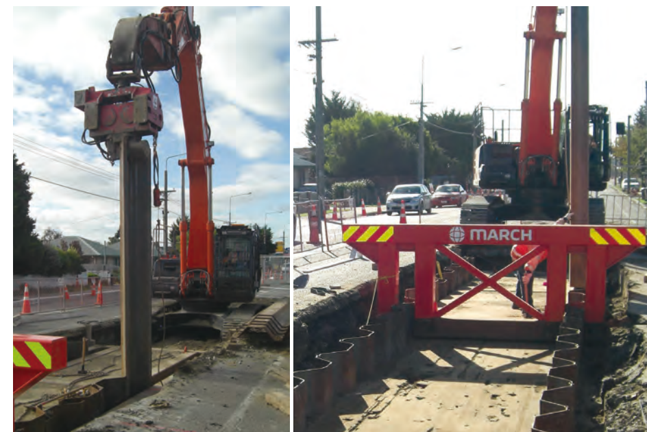
Hat-type Sheet Pile / New Zealand
