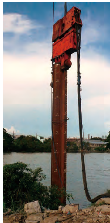
Driving of a Hat+H sheet pile
