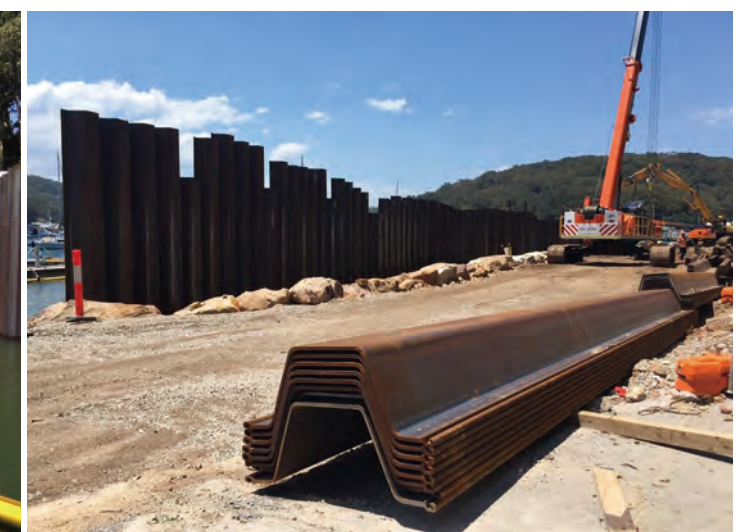
Hat-type Sheet Pile Church point seawall / Australia
