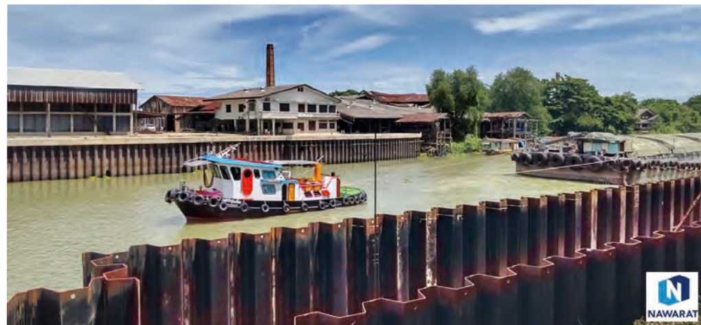
Hat-type Sheet pile River revetment / Thailand
