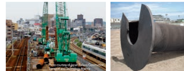
Driving an NS ECO-PILE™ (full-rotation pile driver)
