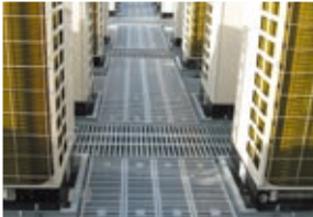
Floors of equipment-related work/inspection platforms
