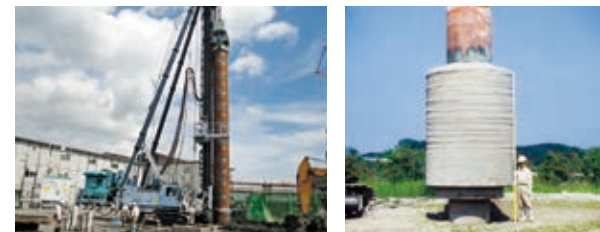
TN-X Method in progress (three-point support type pile driver)
